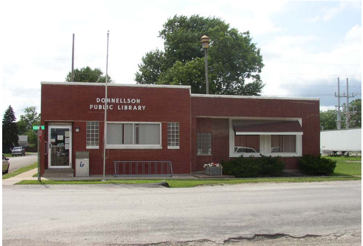
Above: Existing view of the Donnellson Public Library.
